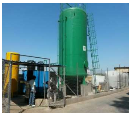
Full scale biogas plant for the treatment of food waste based on AGR at Ahmadabad, Gujarat
