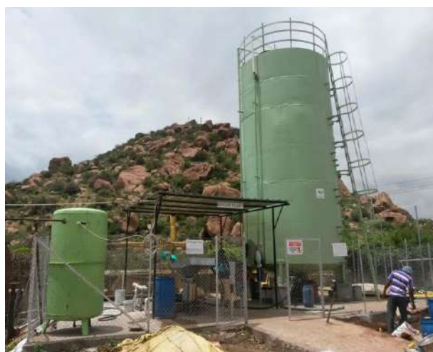
Full scale biogas plant for the treatment of food waste based on AGR at Bellary, Karnataka
