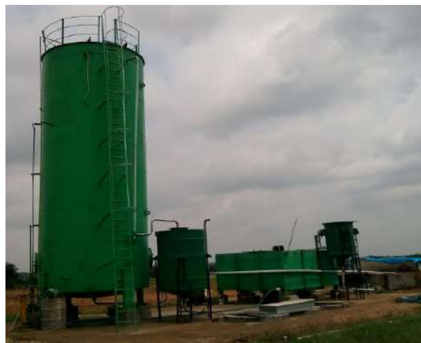
Full scale biogas plant for the treatment of poultry litter based on AGR at Tooparan, Telangana
