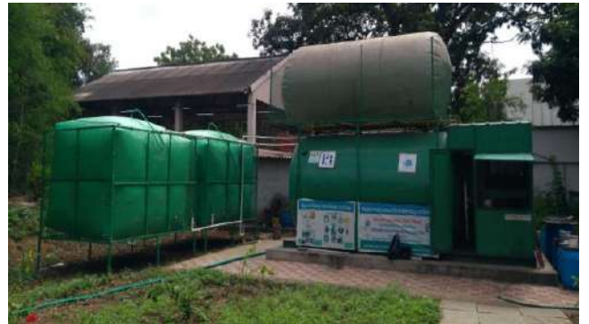
Aerobic Moving Bed Bioreactor (AMBBR) + side stream NF
