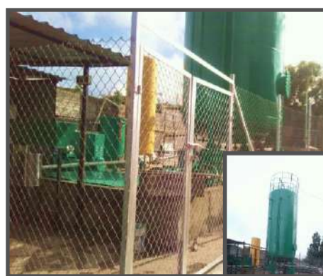
Full scale biogas plant for the treatment of food waste based on AGR at Ahmadabad, Gujarat
